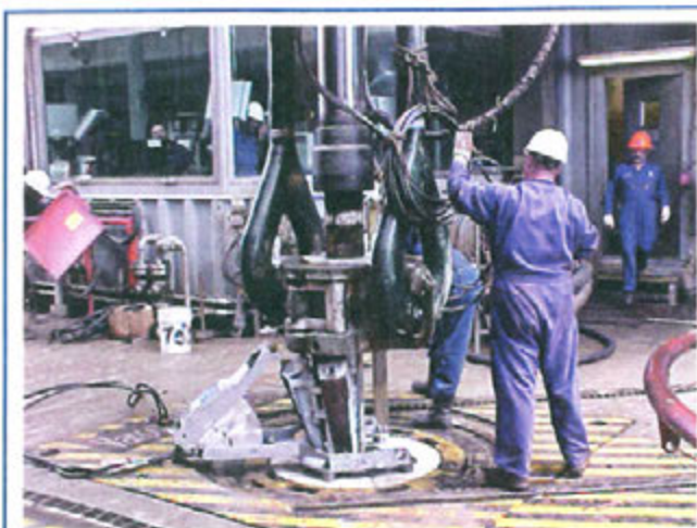
Fig. 5. The new landing string system successfully runs long, heavy casing strings in the 1.5–2-MM lb range.
